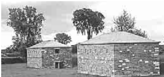
Pictures these two pages: View of the wet ditch, R. Hilborn, Parks Canada, 114/00/PR7/PDO-00027; Ile aux Noix, late 18th century. In the background, the French defence works constructed in 1759 and the British blockhouses erected in 1776, © National Archives of Canada / Capitaine Rudyard / C-40335; Review of the troops at Fort Lennox, © Parks Canada; An aerial view of Fort Lennox today; Rear view of the barracks and casemate, Sophie Grenier / Parks Canada, 114/IN/PR7/SPD-00108; Oil painting by Henry Bunnett, © McCord Museum / Henry Richard S. Bunnett / M-872, 1886; The ordnance magazine and the artillery magazine, Jean Audet / Parks Canada, 114/00/PR7/SPD-00179.
