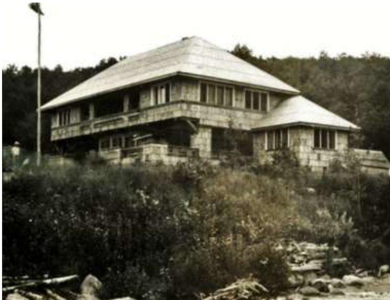
Figure 99 Lismore House under construction, circa 1917-18.
