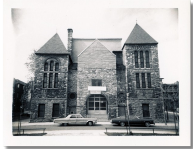
THE NCC (RUE COURSOL, LITTLE BURGUNDY)
