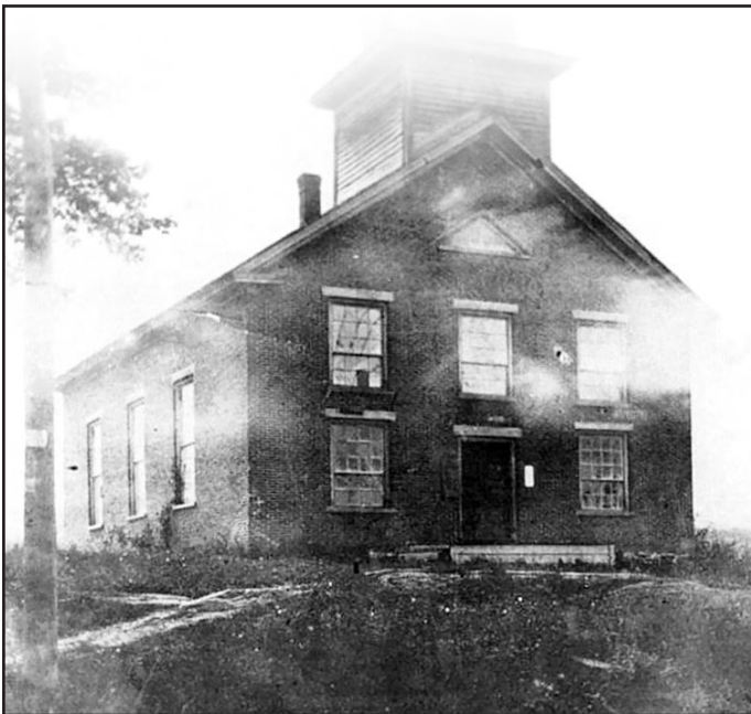
The Baptist church in Mansonville, built in 1847-1848, was sold to the Church of England in 1856. This photo shows the church as Allnatt would have known it. In 1902, this building was demolished and replaced by the current St. Paul's Anglican Church. La Vie dans Potton: patrimoinepotton.org .
