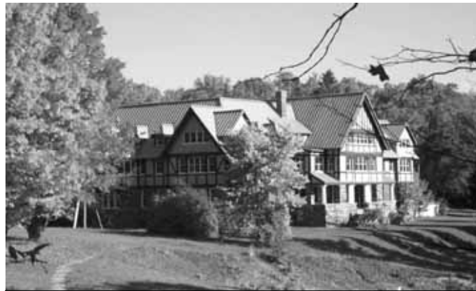
Laurentian Sanitarium. Photo by Joe Graham
