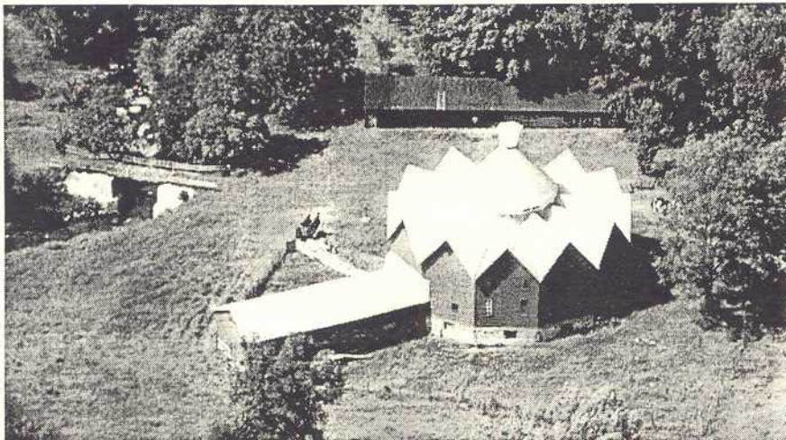
Alexander Walbridge built this twelve-sided barn in Mystic in 1882. It is believed that he modeled it on a railway roundhouse. Photo Hardy Craft
