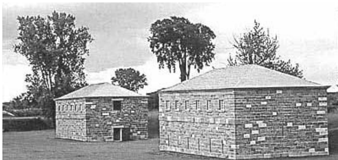
Pictures these two pages: View of the wet ditch, R. Hilborn, Parks Canada, 114/00/PR7/PDO-00027; Ile aux Noix, late 18th century. In the background, the French defence works constructed in 1759 and the British blockhouses erected in 1776, © National Archives of Canada / Capitaine Rudyard / C-40335; Review of the troops at Fort Lennox, © Parks Canada; An aerial view of Fort Lennox today; Rear view of the barracks and casemate, Sophie Grenier / Parks Canada, 114/IN/PR7/SPD-00108; Oil painting by Henry Bunnnett, © McCord Museum / Henry Richard S. Bunnnett / M-872, 1886; The ordnance magazine and the artillery magazine, Jean Audet / Parks Canada, 114/00/PR7/SPD-00179.
