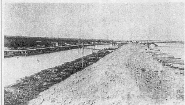
The discharge pipes mounted on pontoons, 5 May 1930
